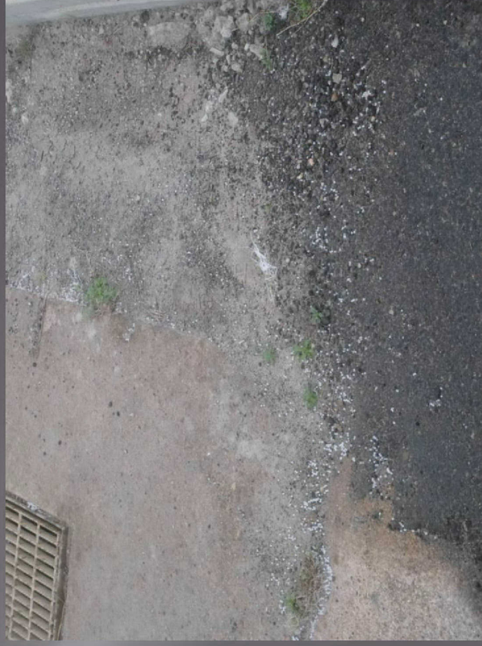
PELLETS LOCATED JUST DOWNSTREAM OF GATE 001.
