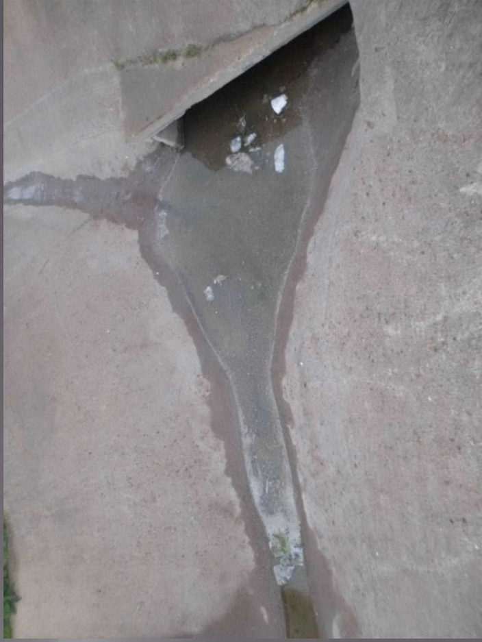
PELLETS AND TRASH ARE VISIBLE IN THIS AREA.
