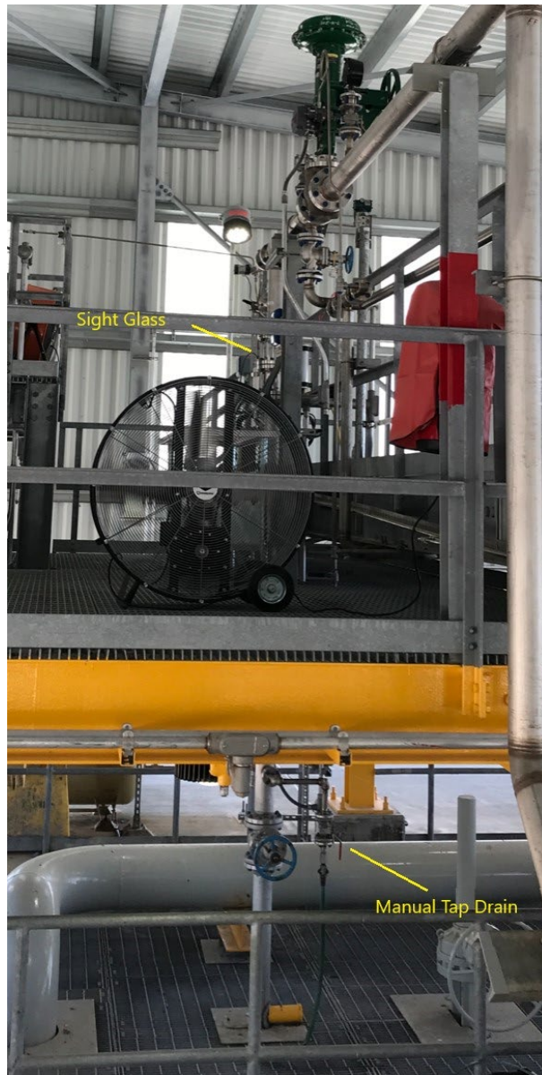
Photograph Z Manual Tap Drain at the WSM to Collect Manual Samples May 31, 2021
