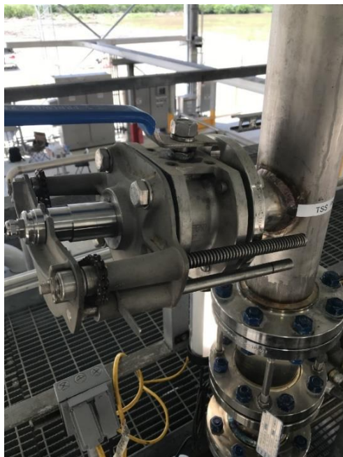
FIGURE 30 – TSS MOUNTING DEVICE
