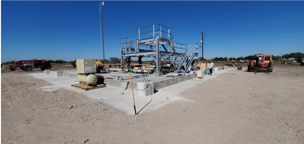
Photograph B Construction of WSM Framing November 17, 2020
