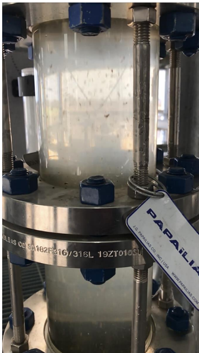
FIGURE 45 - UNACCEPTABLE PRESENCE OF SOLIDS IN SIGHT GLASS, TRIGGERING A MANUAL SAMPLE
