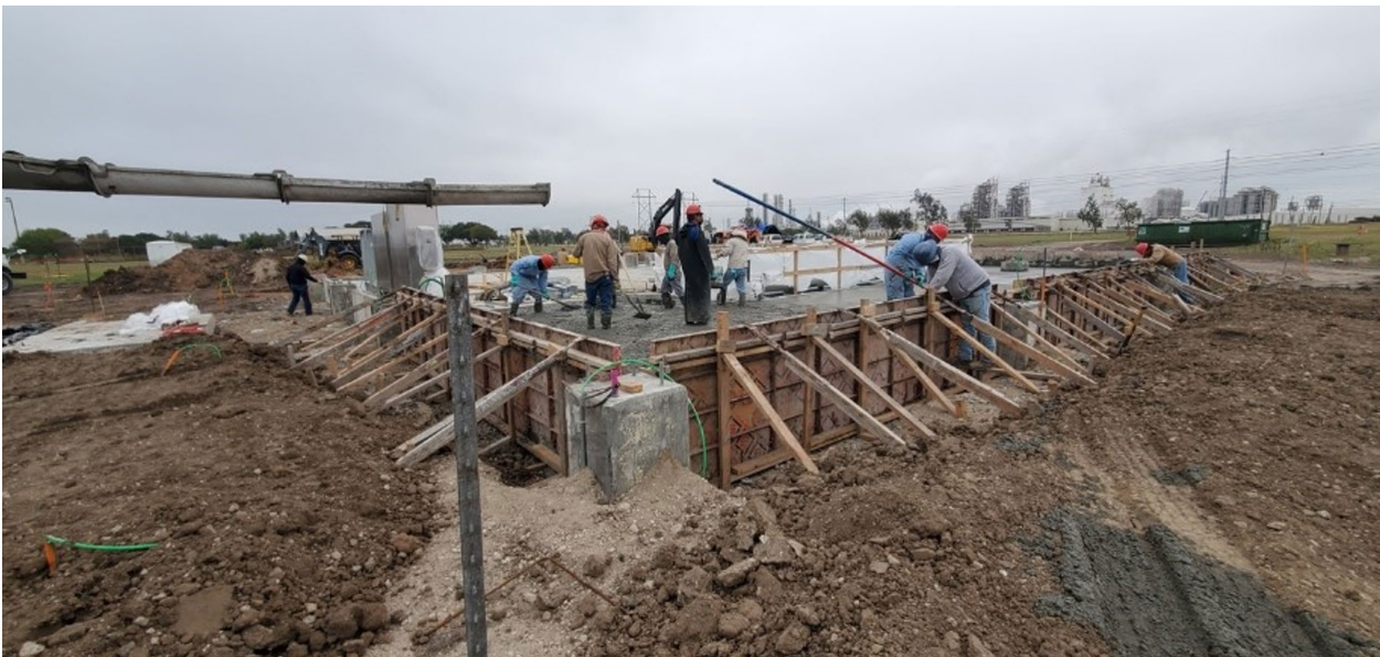
Photograph A Construction of WSM foundation October 27, 2020
