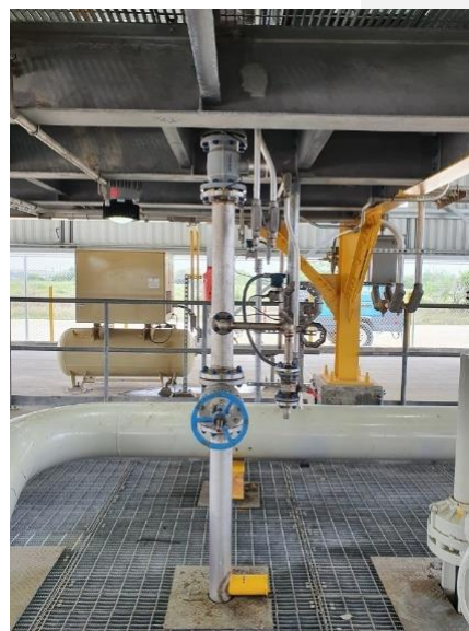
FIGURE 29 – MANUAL TAP DRAIN
