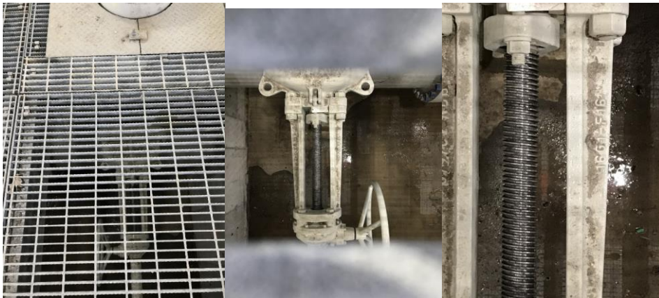
FIGURE 8—BYPASS VALVES CLOSED (COMPLETELY THREADED)
