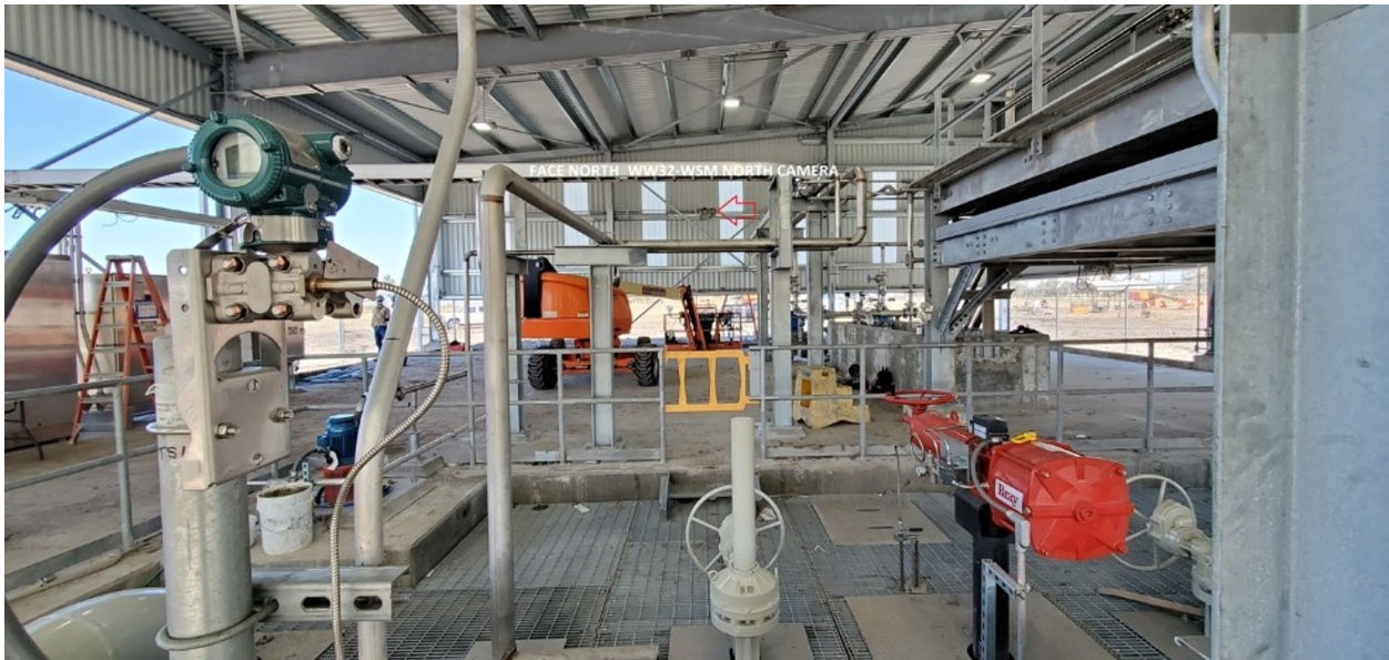
Photograph C Interior Construction of WSM December 28, 2020
