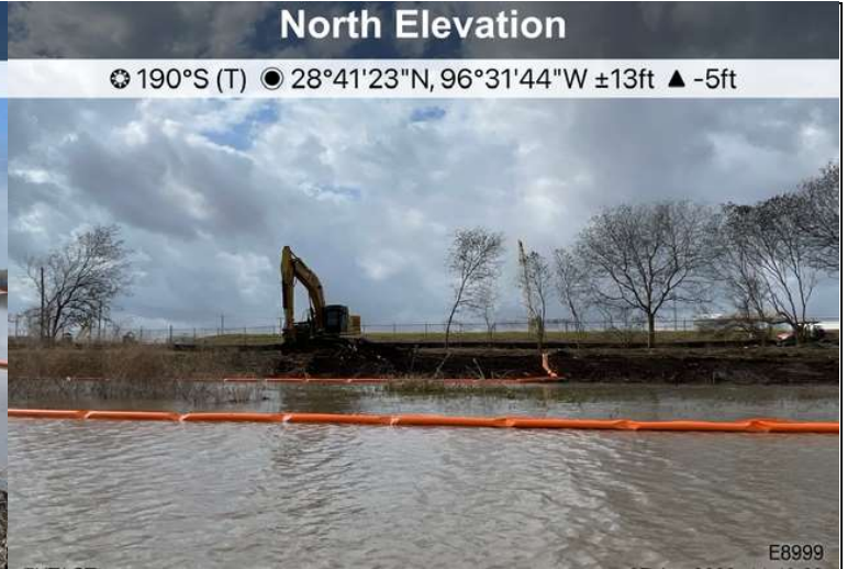
Photo 2. Photo of excavation progress in AOC 17.
