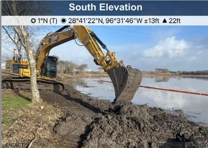
Photo 1. Photo of ENTACT associate performing a 6" removal in AOC 17.
