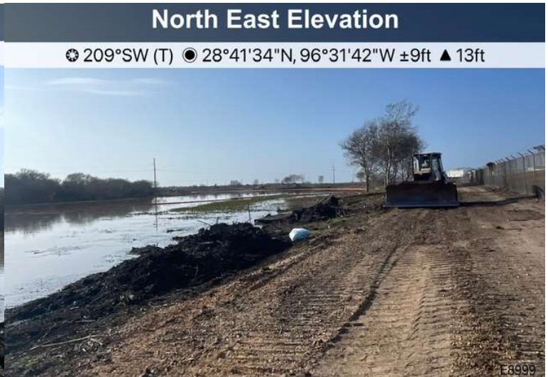
Photo 4. Photo of access road maintenance near AOC 12.
