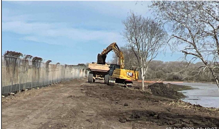
Photo 3. Photo of excavator loading haul truck in AOC 14.
