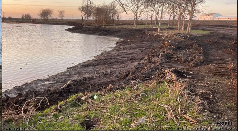
Photo 2. Photo of excavated surface in AOC 14.
